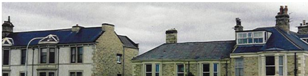
ABOVE: POOR ROOFLINE WORKS - THE ORIGINAL STACK NEAR THE CENTRE OF THE PICTURE HAS NO POTS REMAINING, WHILST OTHER STACKS HAVE BEEN CUT TO LESS THAN HALF THEIR ORIGINAL HEIGHT OR HAVE STUBBY MODERN POTS. A LARGE UNATTRACTIVE DORMER WINDOW HAS BEEN ADDED TO THE ROOF ON THE RIGHT.
