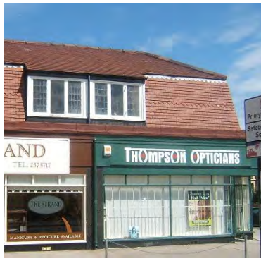
Mansard roof at Queensway
