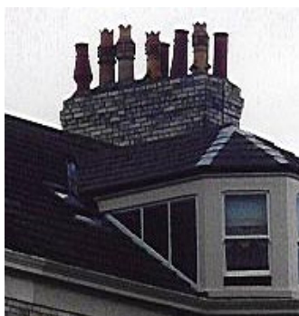
ABOVE: POOR ROOFLINE WORKS - THE ORIGINAL STACK NEAR THE CENTRE OF THE PICTURE HAS NO POTS REMAINING, WHILST OTHER STACKS HAVE BEEN CUT TO LESS THAN HALF THEIR ORIGINAL HEIGHT OR HAVE STUBBY MODERN POTS. A LARGE UNATTRACTIVE DORMER WINDOW HAS BEEN ADDED TO THE ROOF ON THE RIGHT.
